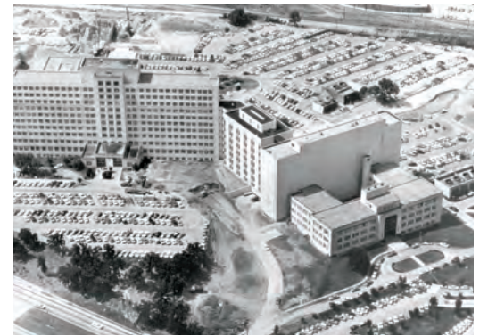
In this photo, circa 1964, Parkland Memorial Hospital is on the left. On the right is the Southwestern Medical School campus, consisting of (left to right) the Danciger (1965), Hoblitzelle (1959), and Cary (1955) Buildings. In the upper left corner is excavation taking place for the building of Children's Medical Center Dallas.
