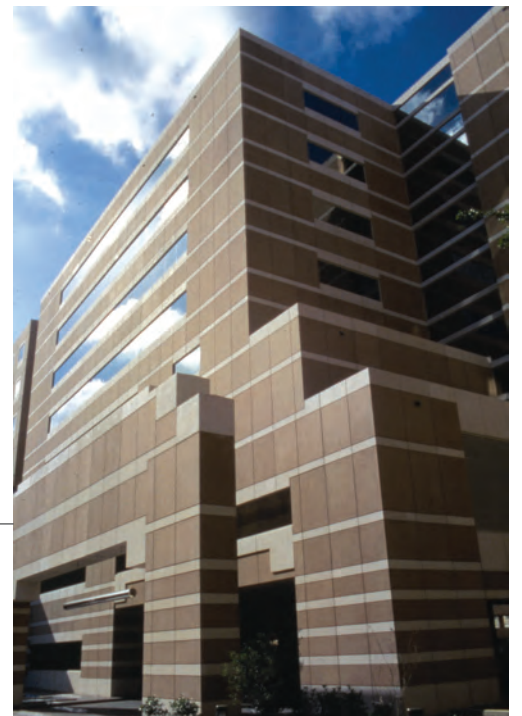
Opened in 1990, UT Southwestern's Charles Cameron Sprague Clinical Science Building houses clinical faculty and also connects with Zale Lipshy University Hospital.
