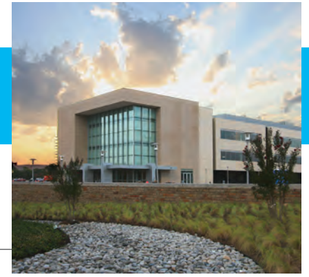
UT Southwestern's BioCenter at Southwestern Medical District was built to provide laboratory and office space to startup biotechnology companies. The BioCenter is located at 2230 Inwood Road in Dallas and opened in the spring of 2010.
